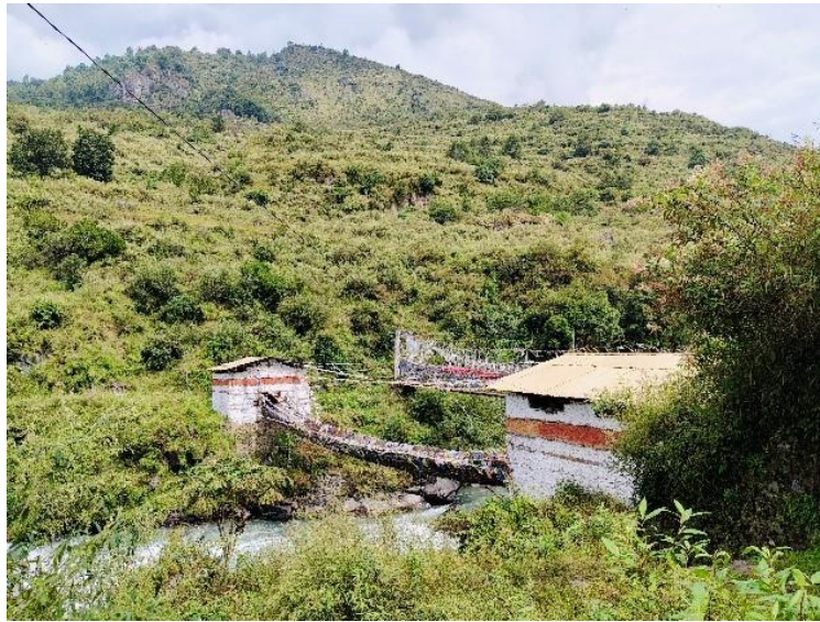
Figure 2. The Chak-zam iron suspension bridge at Tawang River ( chu ) Image: Authors, Tawang, 17 October, 2024
